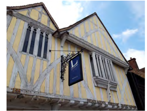
Timber frame of 225 Victoria Avenue with leaded windows and carved cornice
