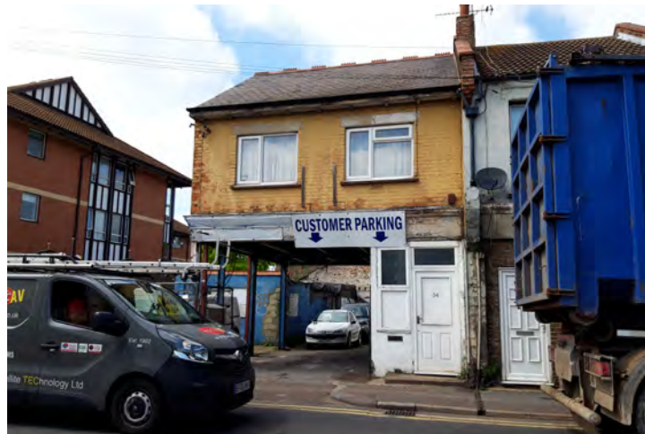
Substantial alterations to this former shop have seriously eroded its historic character
