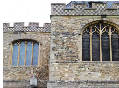
Ragstone church walls with knapped flint chequerboard pattern to crenulations and Gothic windows
