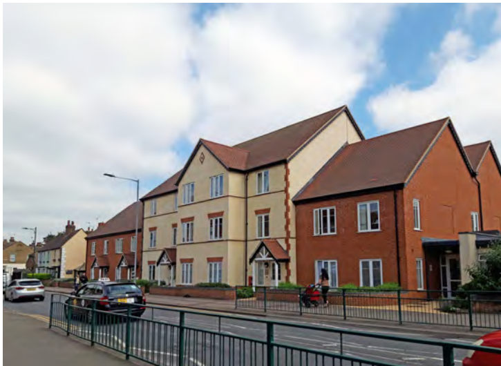
New development in the Conservation Area, of reasonable quality but not contributing to the heritage significance of the area
