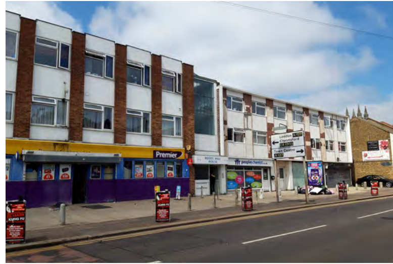
Poor quality 20th century buildings on the north side of West Street with bland forecourt
