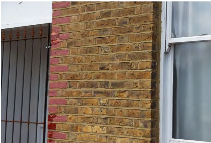
Example of cement pointing to historic brickwork
