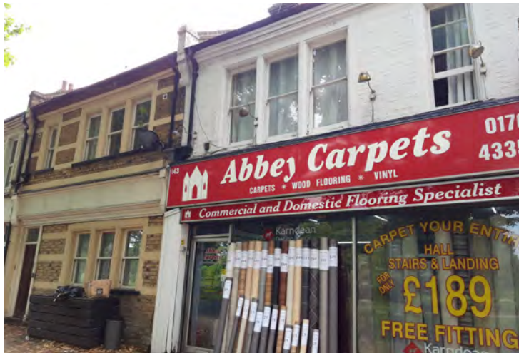
Oversized, garish signage and large area of glazing to a shop front inserted into a terraced house
