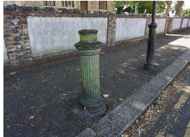
Base of an historic lamppost on St. Mary's road, with modern lamppost base adjacent
