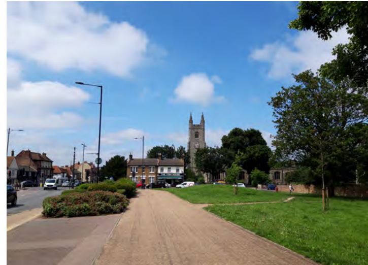
Recent surfacing improvements on the foot/cycleway next to Victoria Avenue
