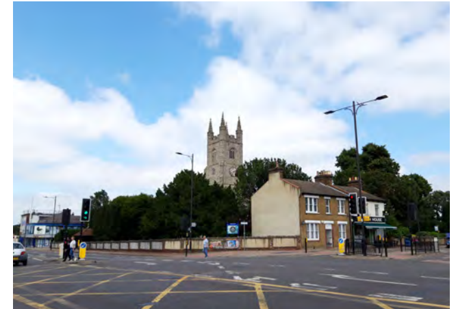
View looking north-east at the crossroads towards the church tower and churchyard
