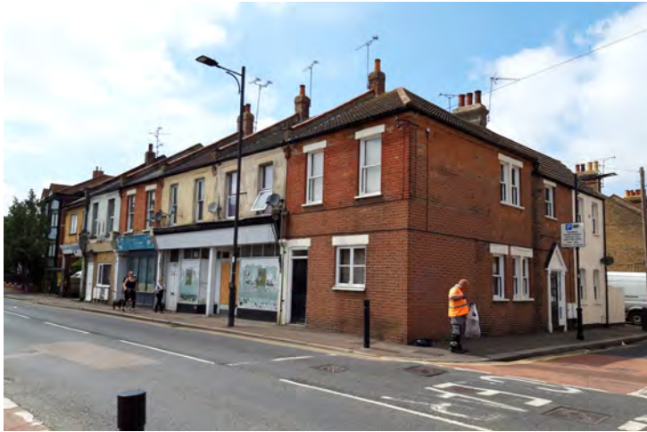
Two shop fronts in this terrace have been converted into residences with windows of an inappropriate scale and proportions for the building. Brickwork has also been rendered and the larger shop is vacant
