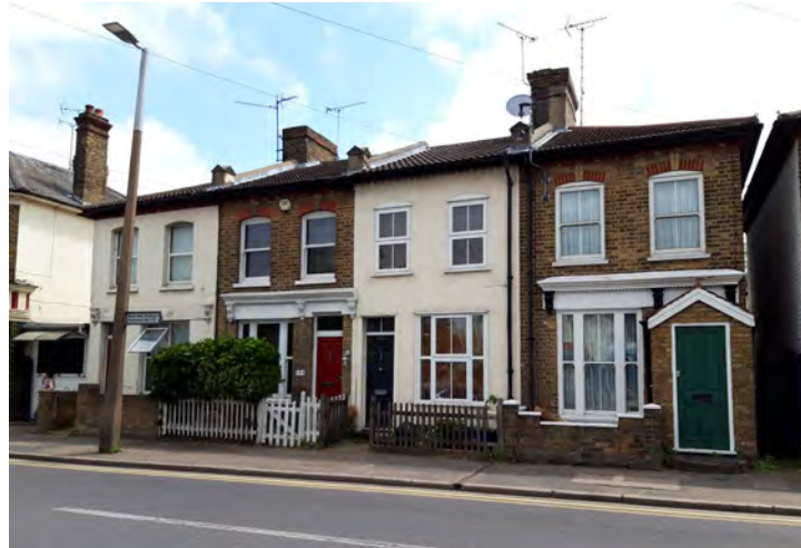
uPVC windows and replacement doors to most of the houses in this terrace. Those in sash form are more appropriate than top hung casements. Two houses have been rendered and have lost their decorative cornices. One has had a porch added.
